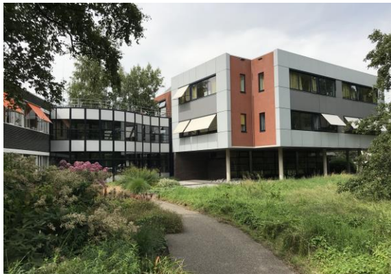
Actual situation before works
